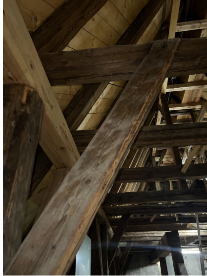
Figure 3: Roof structure of the Dominican Church
