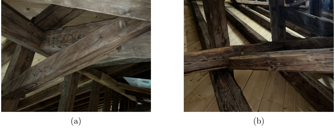
Figure 22: Timber structures captured through the 3D Scanner App for segmentation task
