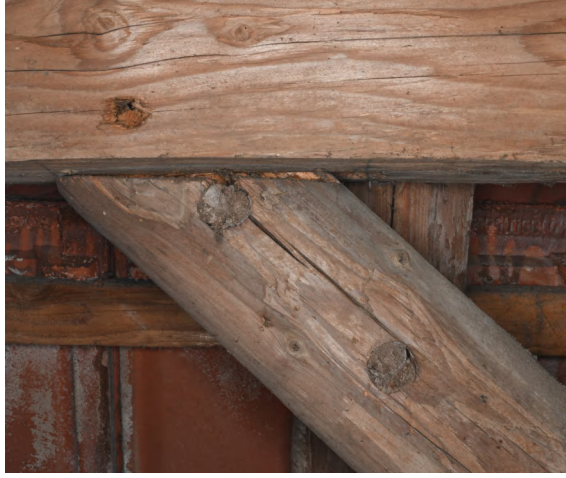
Figure 17: Image captured inside roof structure in Schweinfurt
