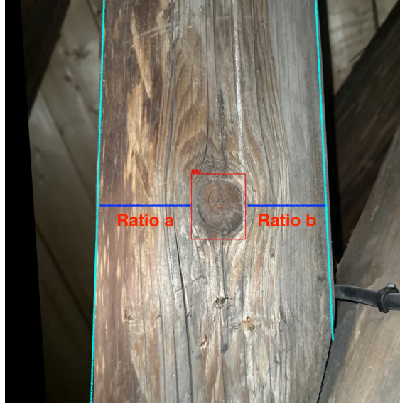
Figure 69: Schematic explanation of the ratio export based on the size and position of the detected bounding box and the perspectively corrected polygon of the timber boundary
