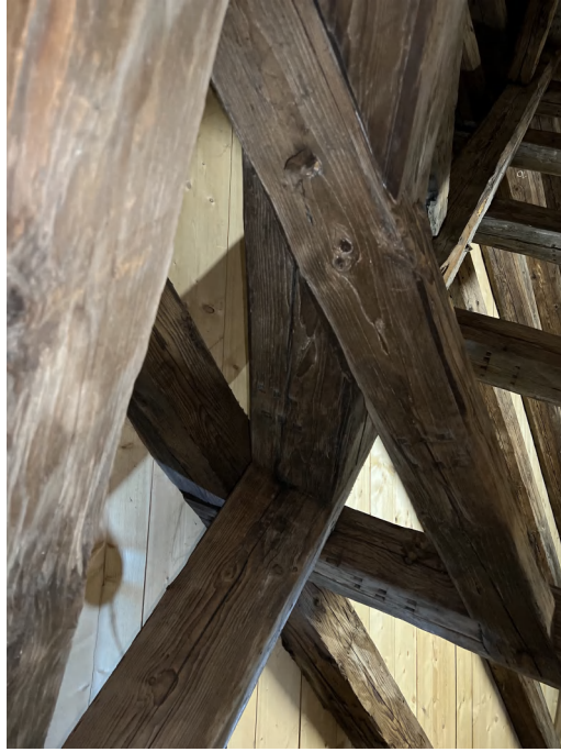
Figure 18: Roof structure of the Dominican Church
