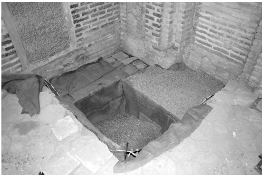
Golpayegan, Friday Mosque: Filling of trenches after documentation
